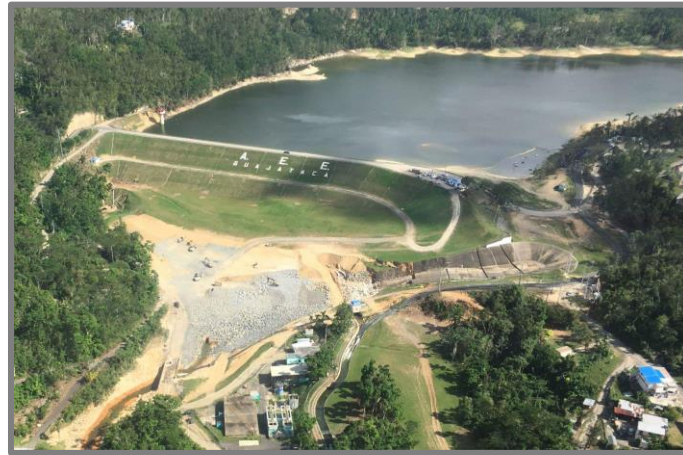
Figure 6: Guajataca Dam (photo by US Army Corps of Engineers)
