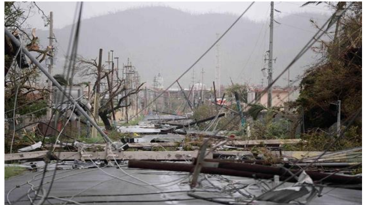
Figure 9. Hurricane Maria Damages Year 2017
